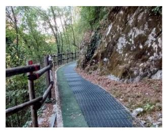
The bottom is now on a metal grating, below which we can see the original channel of the abandoned pipeline.
