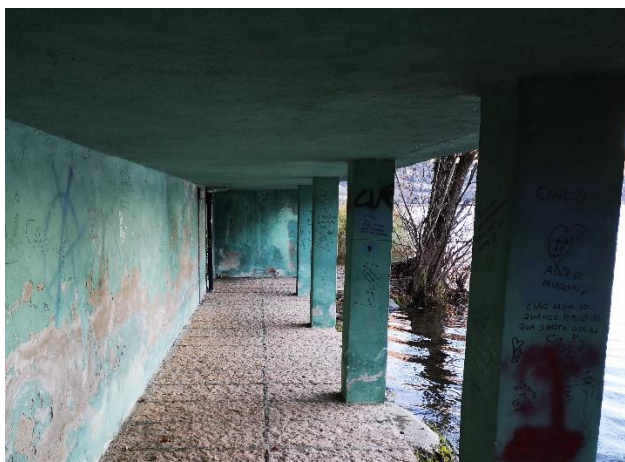
The surface consists of cement and stone rectangles, and the height from the ground is low.
