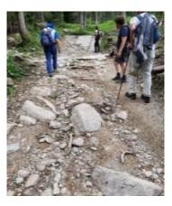
Even very uneven stretches with partially cemented sections and others with stones embedded in concrete screed. The width of the route is constant at around 3 metres.
