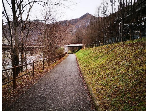
Continuing along we meet a bridge that joins the two San Pellegrino plants.
